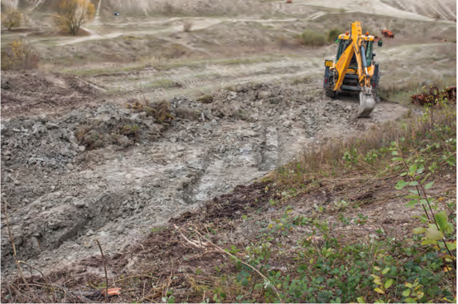
Plate 6. Creation of shallow seepage pools at Sundon quarry using a mechanical digger to strip away the top soil first and then form a herringbone pattern of pools.
